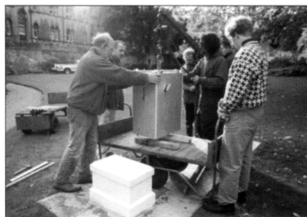
Fig.6 Hoisting the main dial with the lewis pin. The wood protective cladding is still on the dial. The Meadows Building is in the background.
